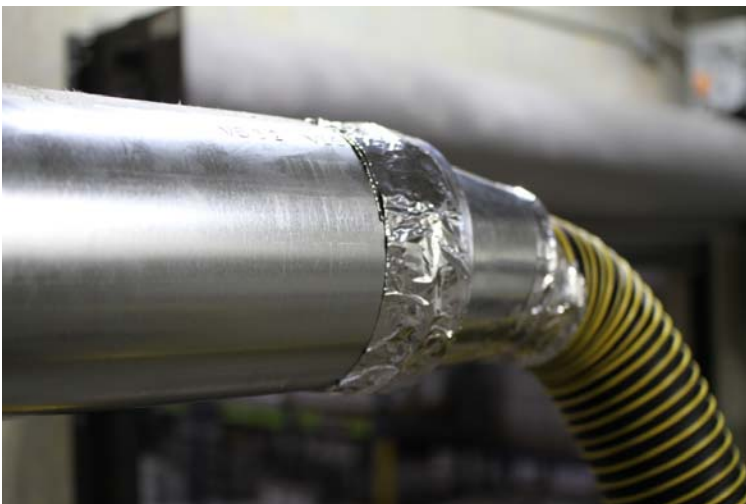
Figure 6 – Connection to Duct System
