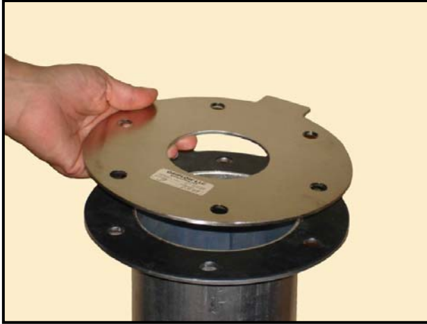
Figure 1 – Installing Orifice Plate
