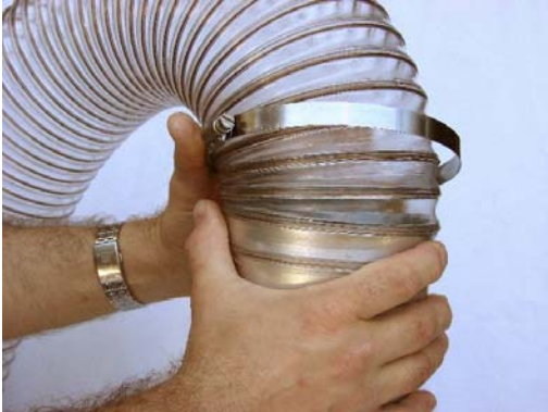
Figure 4 – Installing Flex-Duct on Tube
