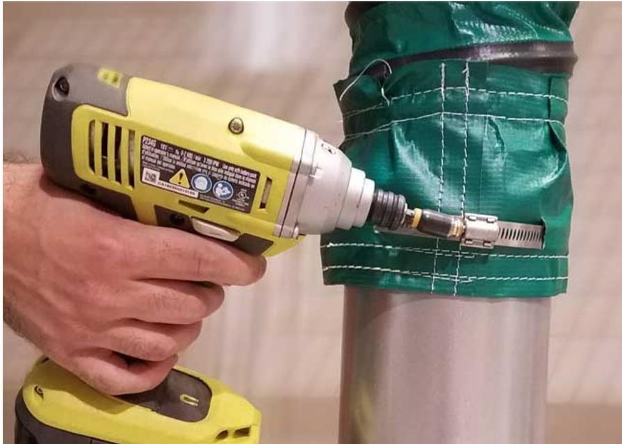
**Figure 5** – Installing Flex-Duct on Tube
