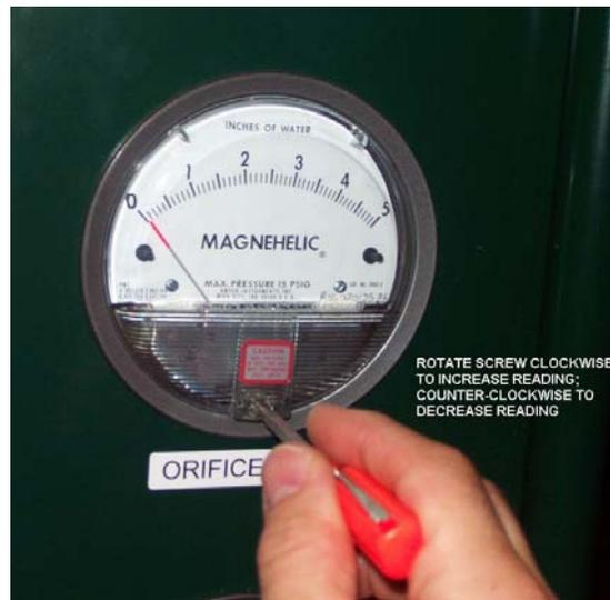
**Figure 10** – Zeroing Analog Gauges
