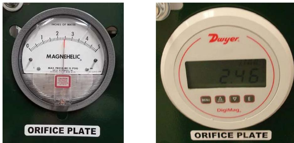
**Figure 14** – Orifice Plate Pressure Drop (analog on left, digital on right)
