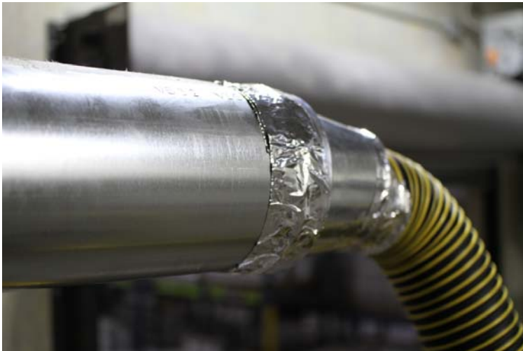
Figure 7 – Connection to Duct System
