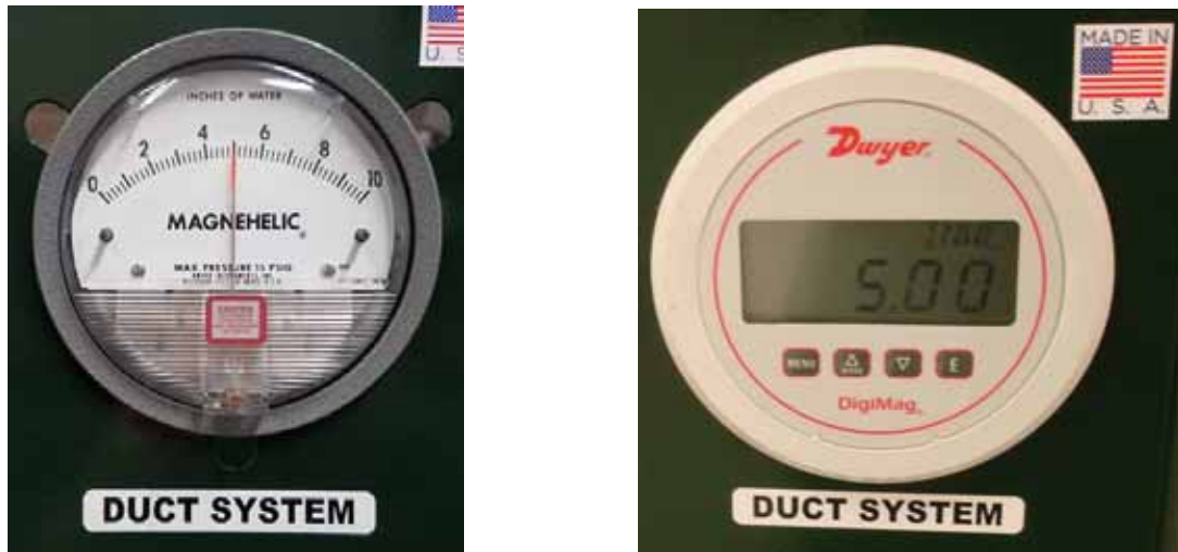
Figure 13 – Duct System Gauge Reading (analog on left, digital on right)
