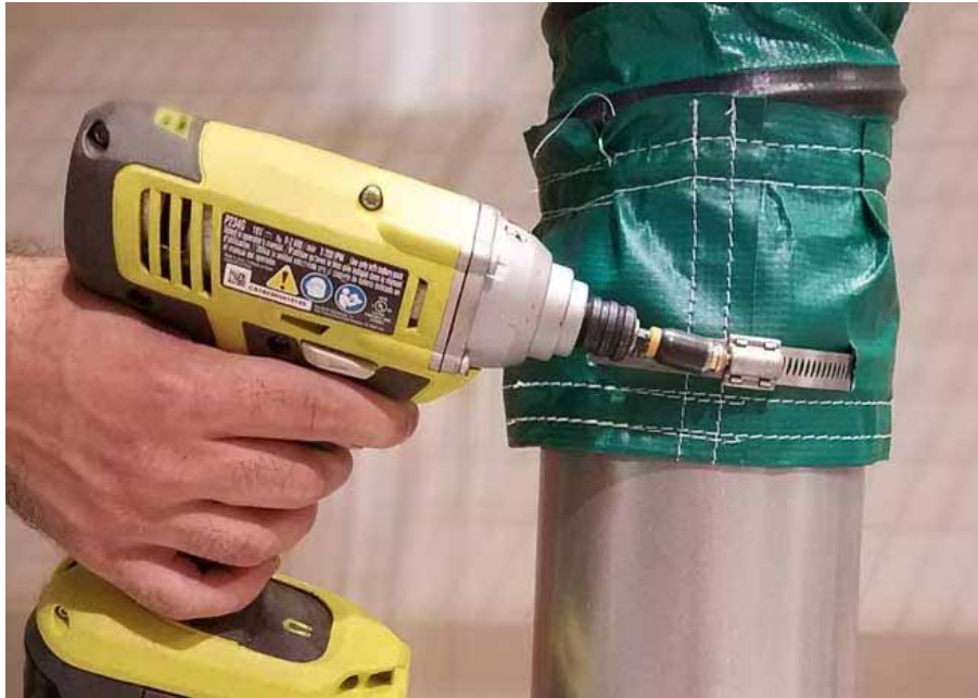
Figure 5 – Installing Flex-Duct on Tube
