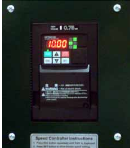
Figure 11 – Avoid Over-Pressurizing by Minimizing Air Delivery upon Startup (inlet slide model on left, VFD speed control model on right)
