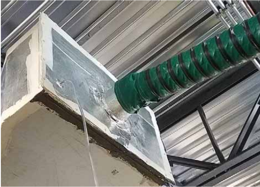
Figure 6 – Connection to Duct System
