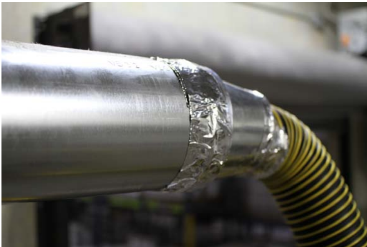
Figure 6 – Connection to Duct System
