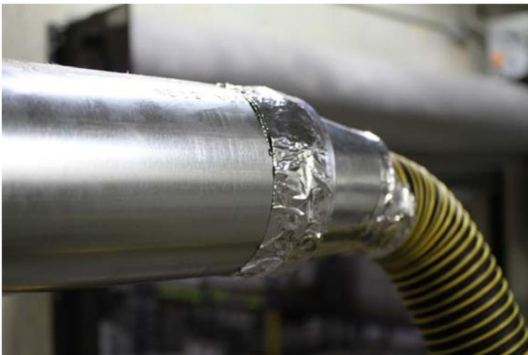
**Figure 6** – Connection to Duct System
