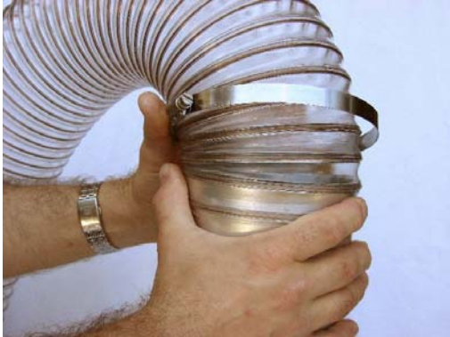
Figure 4 – Installing Flex-Duct on Tube
